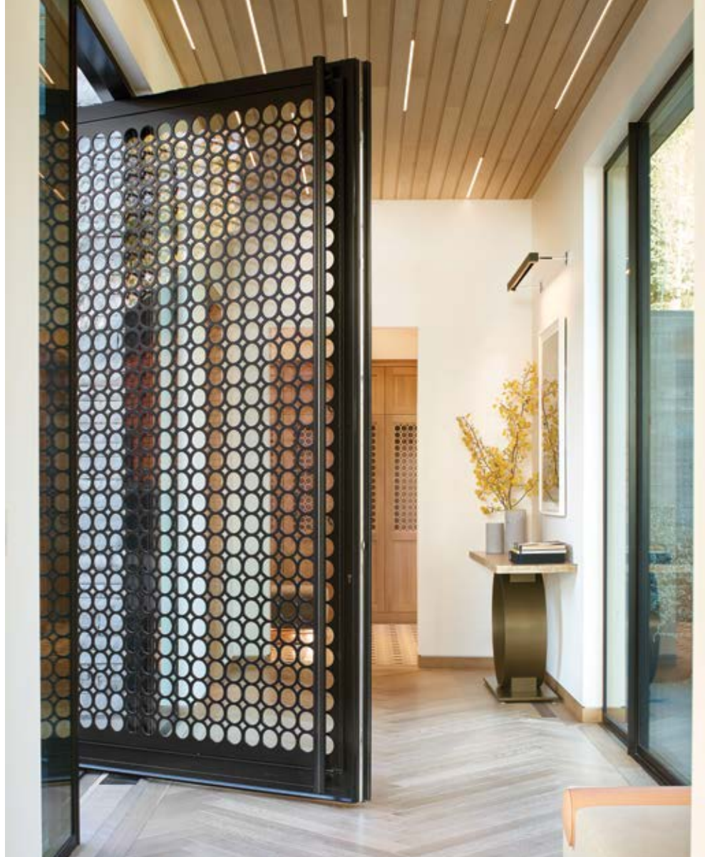
« Entry Door Architect Kyle Webb designed the front door to capitalize on the spectacular view beyond the entrance. The door is made of steel with laser-cut patterning and was manufactured in Italy by Brombal. Trimworx installed the white-oak ceiling.
